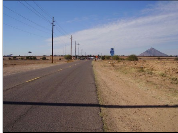
Typical ADOT overpass (0.25 mile away)
