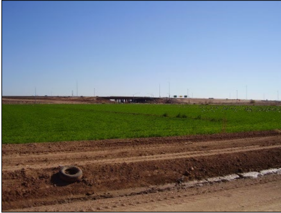
Typical ADOT overpass (0.25 mile away)
